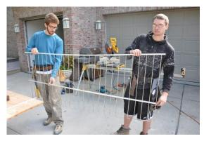
8) "DROP" After the "Hook" now the "Drop". Just let the bottom support channel fall freely to the bottom while still holding on to the top channel creating the infill.
