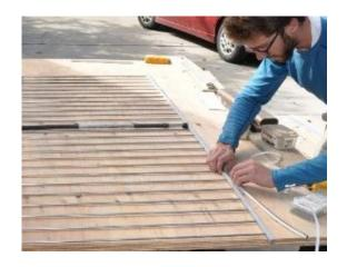
9) Peel the tape off rubber damper and push the sticky side into the channel pressing as you go. Adhesive is only temporary to hold rubber until Invis-A-Rail is attached to your rail system. (TIP: Best assembled on a 4x8 sheathing on horses as a table.)
