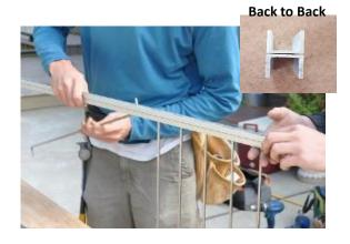
7) "HOOK" Hold support channels back-to-back and aligning holes, hold about chest high. Feed the balusters in from the bottom side hooking in place. Longer length rails above 5ft may be easier with an assistant. (TIP: Keep balusters facing the same direction.)
